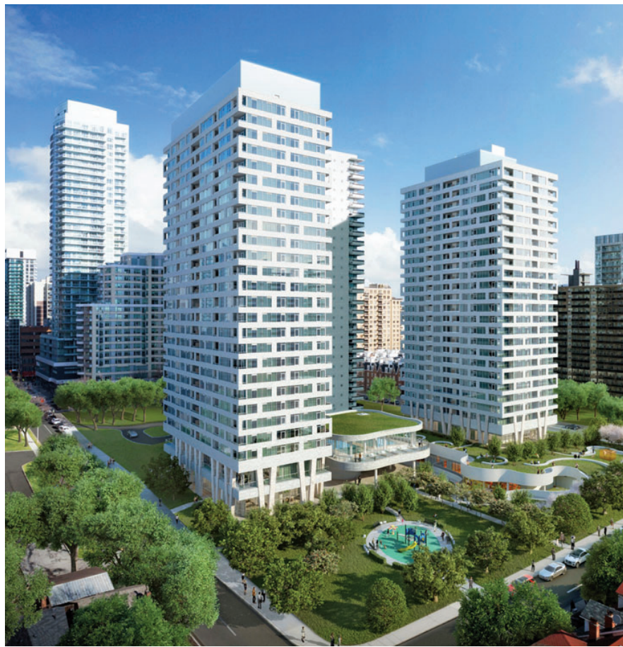
Geothermal heating and cooling are being used in some very large projects. This is an artist's concept of a 542-unit condo complex currently under construction in Toronto.
